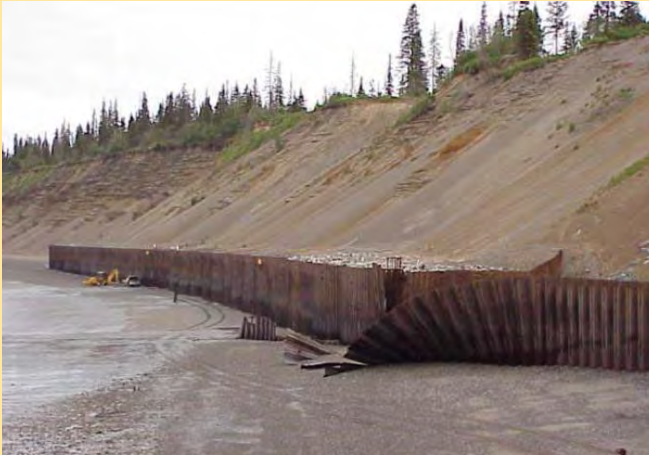
Metal Sheet Piling Fence
