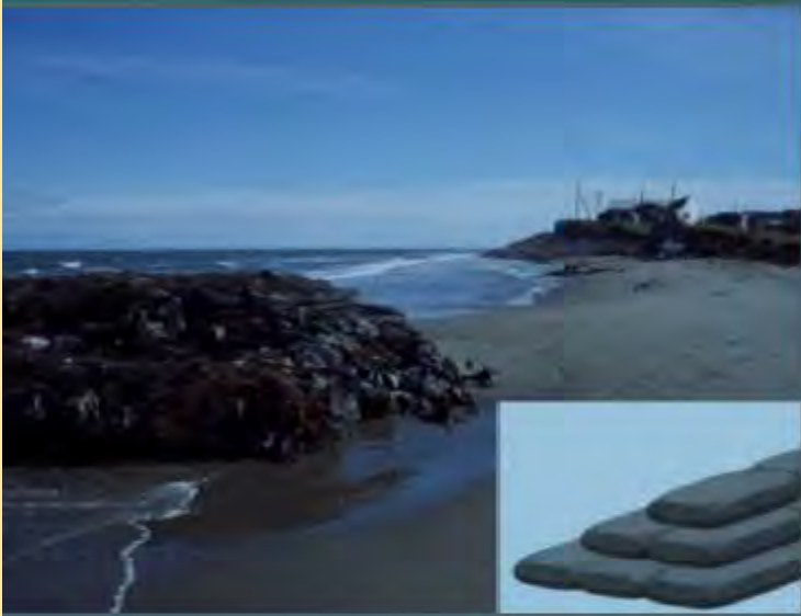
(a) Concrete Filled Bags
